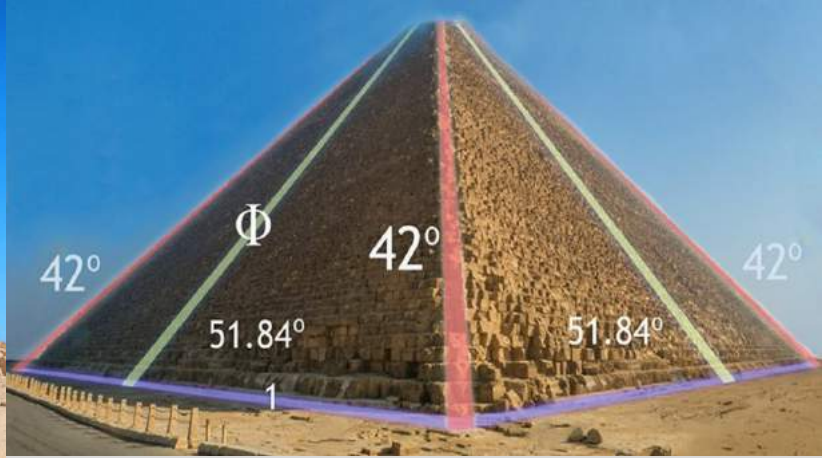
Gambar 2. The Great Pyramid's slope angles. Sumber: Dergice.
